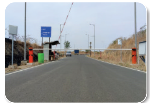
Execution of PGMS - Booking Software, CCTV cameras, RFID Based Boom Barrier, Weather Monitoring Station, On Board Navigation unit
